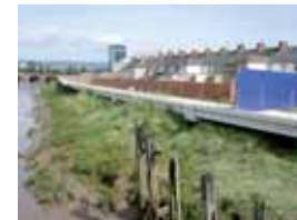
Colne Street: after
