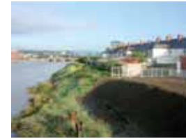
Colne Street: before
